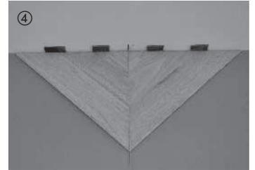
First, fit together three left and three right elements without adhesive to form a "head". Align it with a chalk line. Measure the distances to the wall and cut the elements accordingly. The leftover pieces can be used on the other end of the braid. The chalk line (centre of picture) runs exactly through the centre of the room. The number of rows is determined from the room's width divided by the covered width (523 mm) of an element (see Fig. 1).
