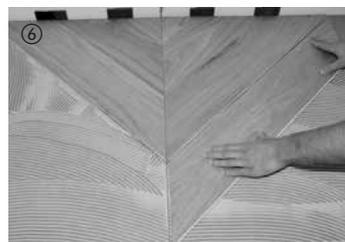
The short-side layer strips run exactly under the chalk line. Glue down the first Chevron row (braid) along the chalk line. Make sure that the tops fit exactly together and that all joints are closed.
