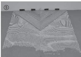
Apply adhesive with the Hamberger special spreader D along the chalk line laid out in the centre. The width of the adhesive application equals the width of a covered width to the left and the right of the chalk line. Lay the boards previously laid out and fitted together into the glue layer. Only apply adhesive for the area you can install in 15 minutes.
