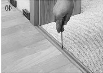
Leave an expansion space of approx. 5 mm between the board and the base of the moulding. As a rule, a fine saw must be used to cut a gap the thickness of a board in wooden door frames to allow the laminate floor to expand. Be sure to remove all distance spacers once all boards are laid. Fasten skirtings (with or without clip system) to the walls -- that's it.
