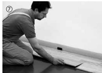
⑦ The next row is started with the leftover piece of the first row (short side offset of at least 50 cm). This considerably reduces waste. The rest of the installation is performed board-by-board. First, the boards are angled into the previous row along the long side by applying a small amount of force.
